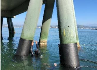
ENVIRAWRAP is an elastic, multilayer, polymer wrap applicable by induced tension. It allows to perform a durable corrosion protection of risers for offshore platforms, piles of harbor piers, jetties, offshore wind farms and operating water pipeline's field joints; enabling rapid operations (for both installation and inspection), requiring minimal substrate preparation and without the aid of flames or particular tools.
